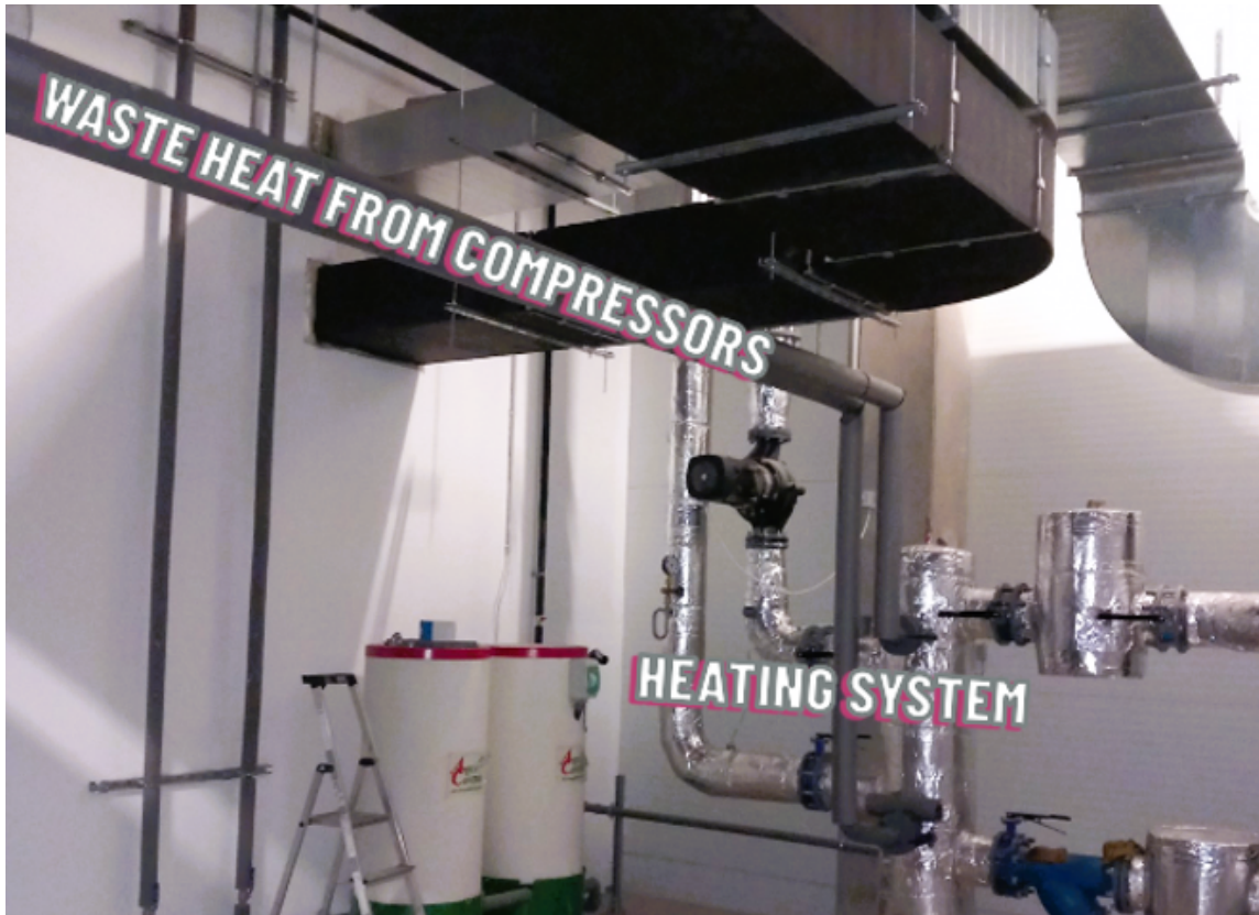
Compressor waste heat recovery in our Hungarina plant
